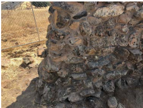
Mortar applied to sign edge to fill gaps, and reinforce missing stone photo credit EDH Save Our Sign
