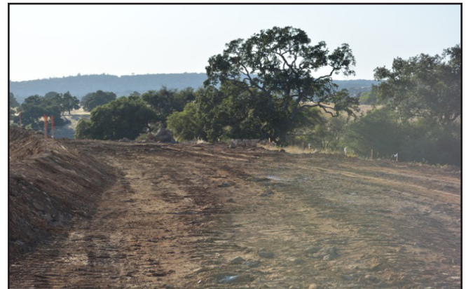
Looking downhill towards Bass Lake Road and the new intersection.
