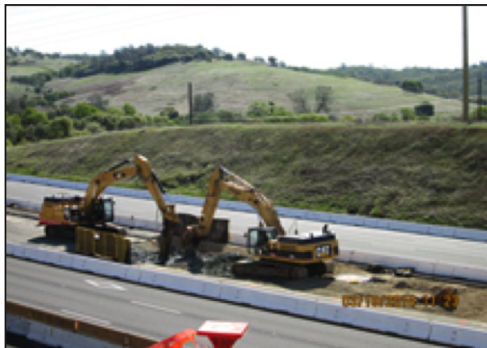
Vainly trying to excavate the foundation for the center median supports for the Silva Valley overpass in the solid rock.
