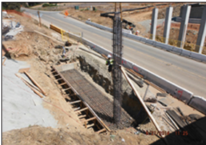
Fabricating the overpass supports for the ramp that will cross Old Silva Valley Parkway on the north side of Highway 50.
