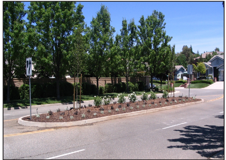
Finished median showing the new landscaping of ornamental pear trees, roses, loropetalum and society garlic
