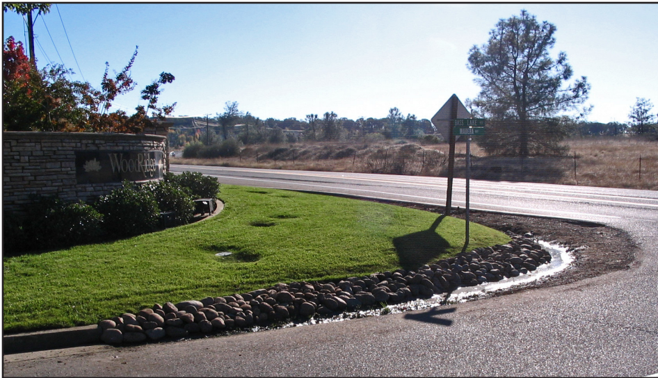
One corner of the intersection showing the drainage improvements
