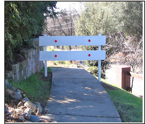
New end-of-sidewalk barrier
