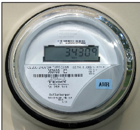
Typical smart electric meter
