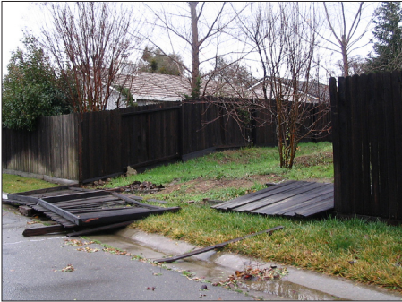
Examples of fence damage from recent wind and rain storms
