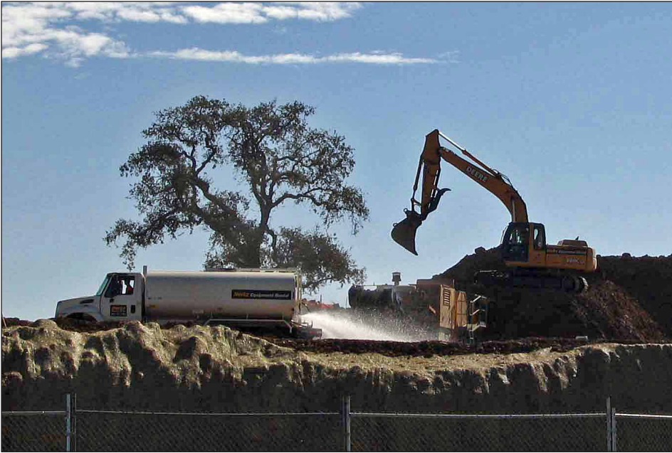
Grading operations at Montano de El Dorado
