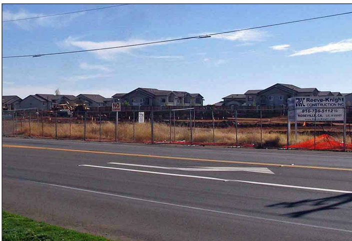
Green Valley Station in progress
