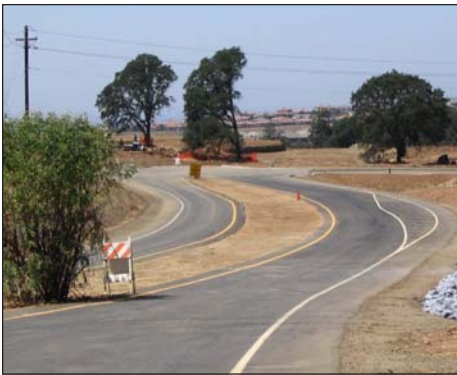
Part of the new Bass Lake Road link
