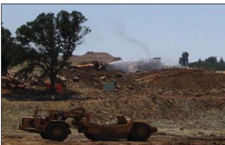
Construction on the realigned Road
