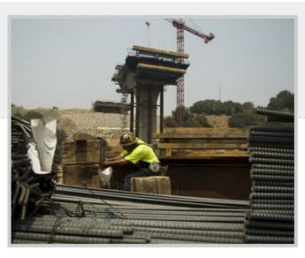
Mark Soulie, an ironworker on the Folsom Lake Crossing bridge project, ties together steel bars that will go in place as the center span is built.
