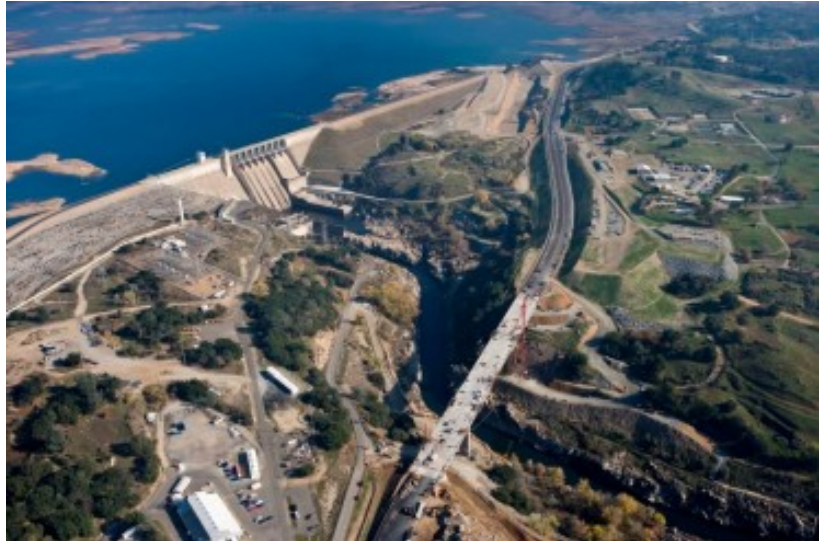
Folsom Lake Crossing is shown in this December 2008 file photo supplied by the city of Folsom. The bridge is slated to open March 28.
